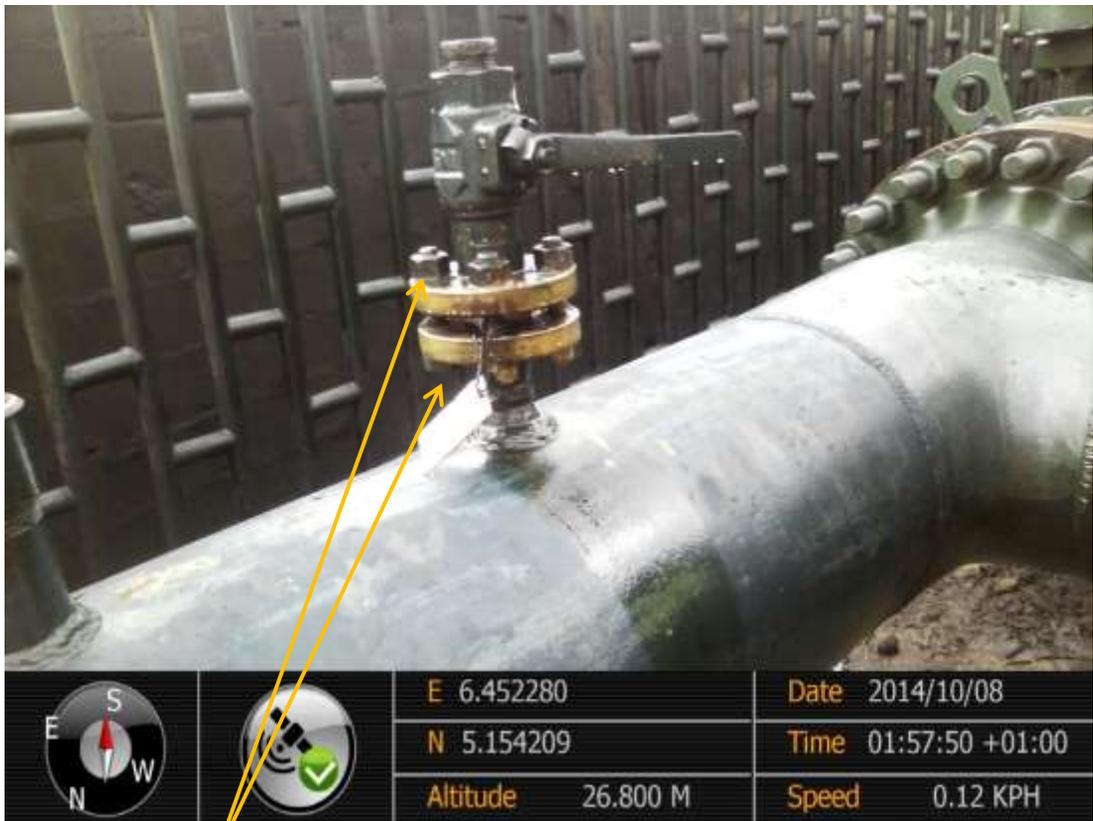
Close-up: Tampered flange nuts on Okordia Manifold at Ikarama. Picture was taken during Joint Investigation of 8<sup>th</sup> October 2014.
