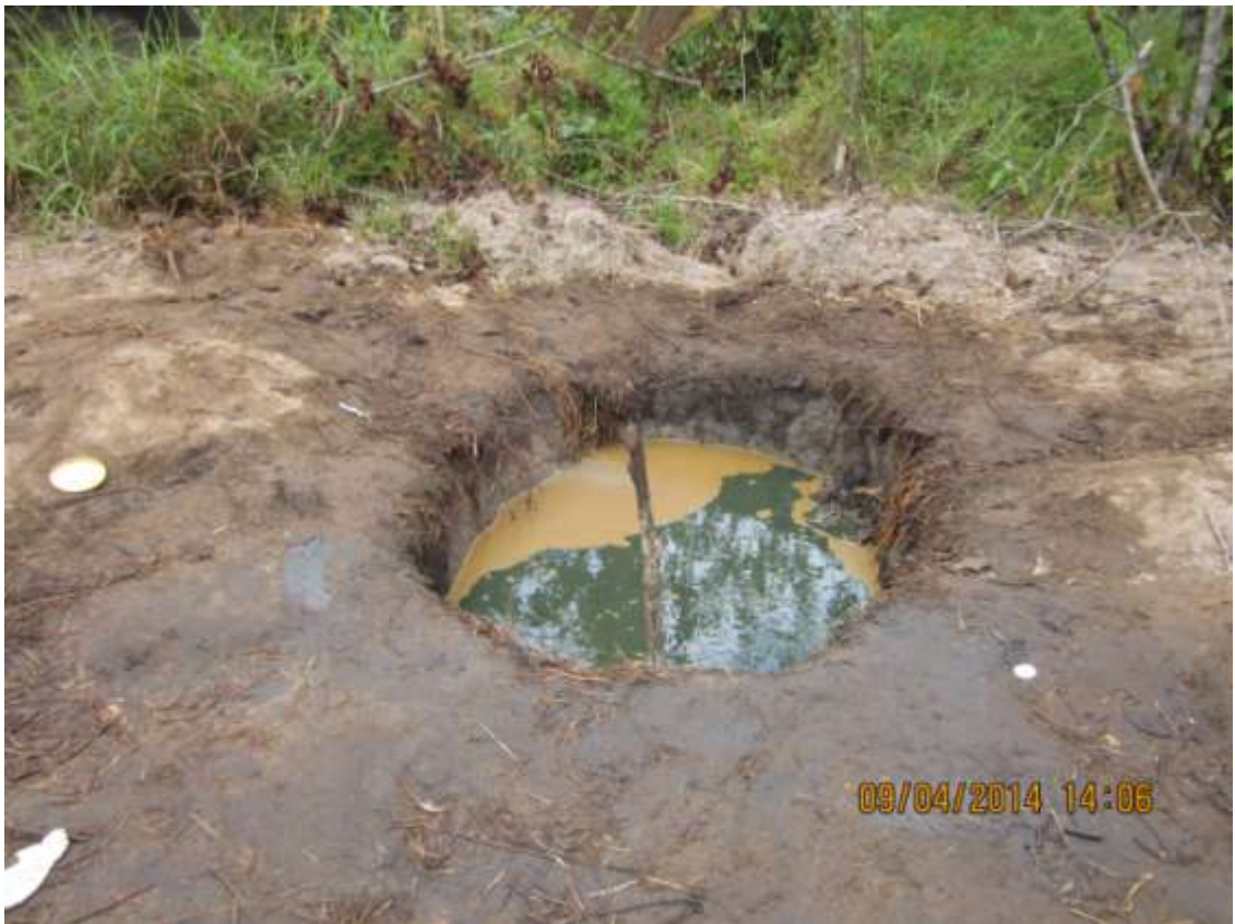
Overview: Part of spill impact on 20" Rumuekpe – Nkpoku Pipeline right of way at Omusunu/Ibaa. Picture was taken during Joint Investigation of 9 th April 2014.
