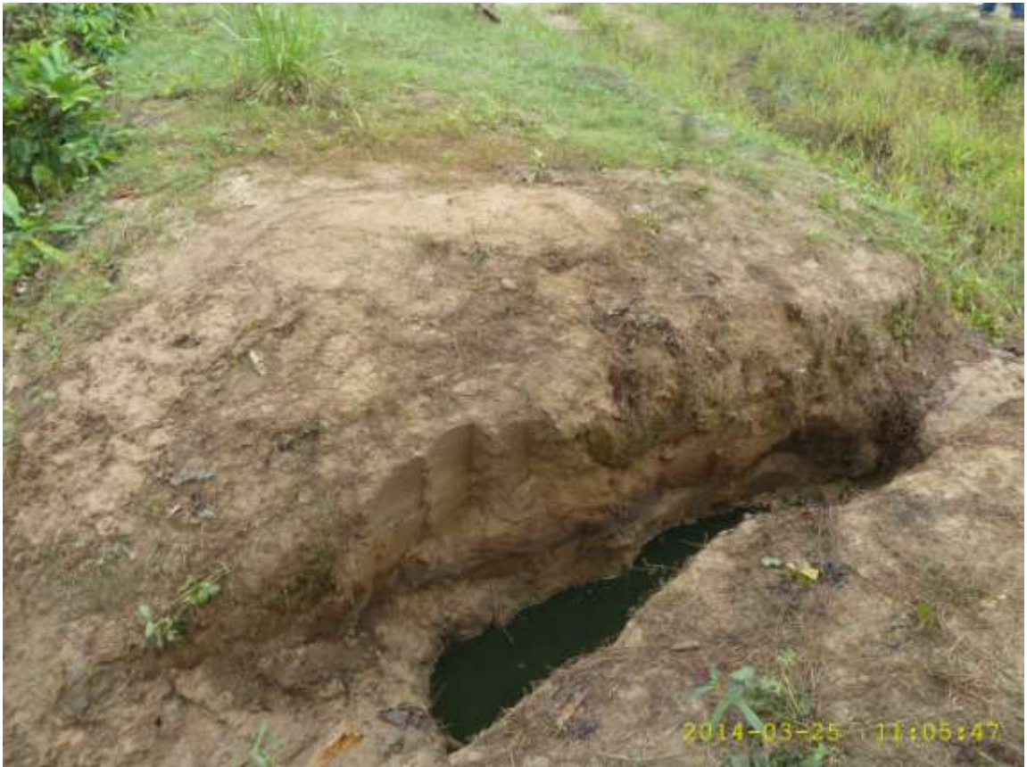
Overview: Part of spill impact on 28" Nkpoku-Bomu Pipeline right of way at Kpoghor. Picture was taken during Joint Investigation of 25 th March 2014.
