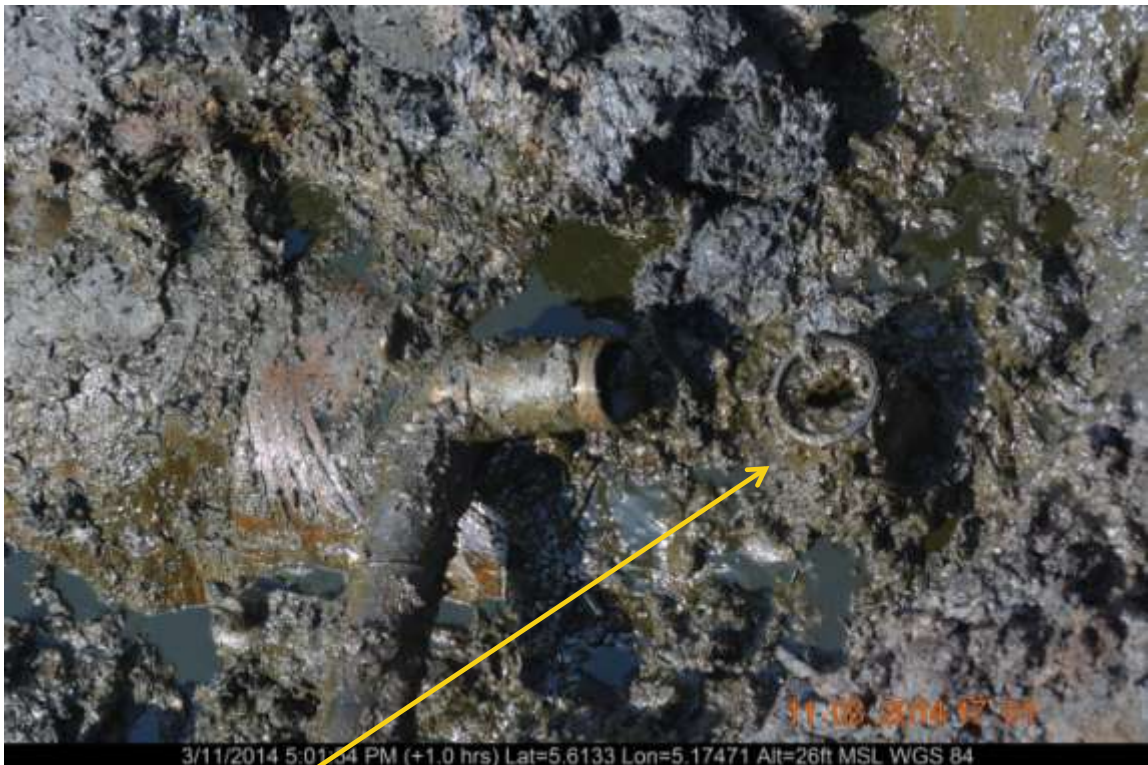
Close-up: Illegal fitting on 20" Otumara-Escavos Pipeline at Ugboegungun. Picture was taken during Joint Investigation of 11th March 2014.
