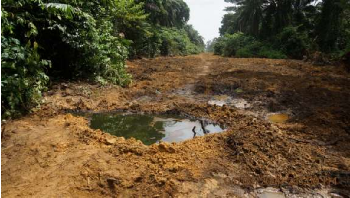
Overview: Part of spill impact on 20" Otumara-Escravos Pipeline right of way at Adjudaibo. Picture was taken during Joint Investigation of 4th March 2014.
