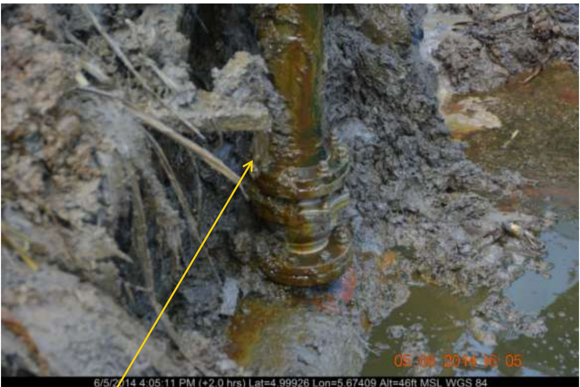
Close-up: Illegal fitting on Benisede – Brass Creek Pipeline at Ojobo. Picture was taken during Joint Investigation of 5 th June 2014.
