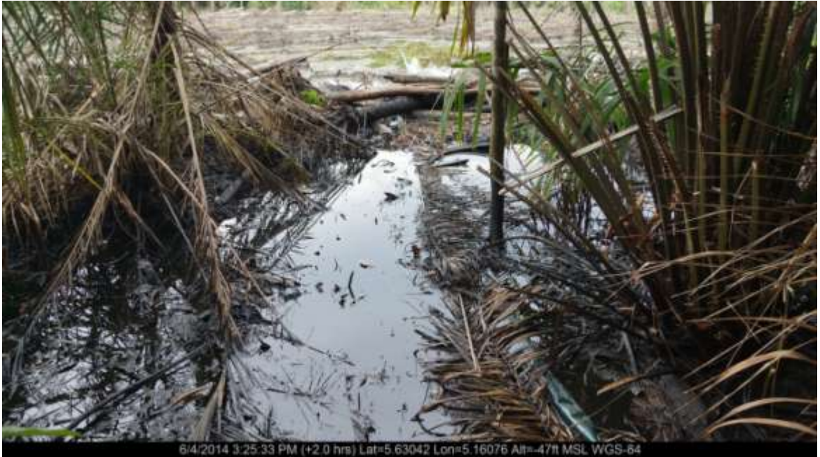
Overview: Part of spill impact on 20" Otumara – Escravos Pipeline Right of Way at Ugboegungun. Picture was taken during Joint Investigation of 4 th June 2014.
