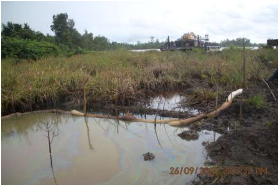
Overview: Part of spill impact on Kanbo Well7S flowline right of way at Egbemoangarabiri/Agbidiama.
