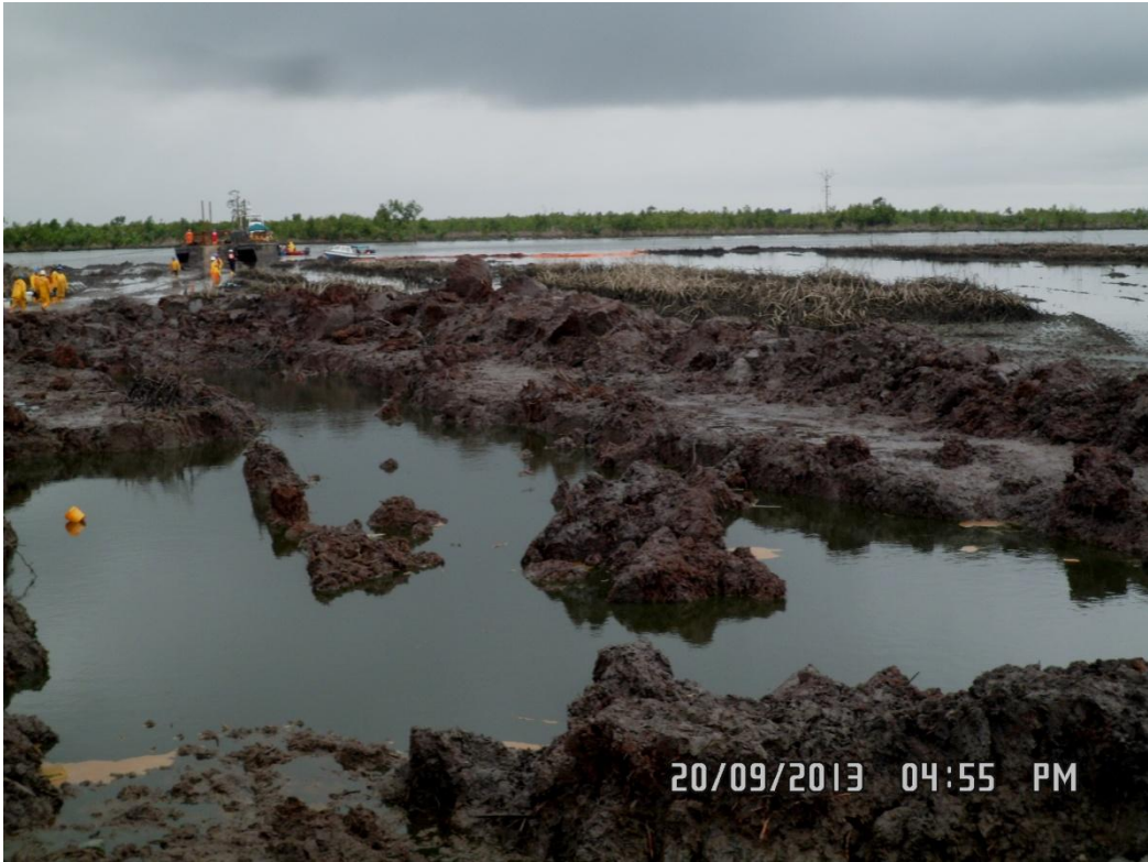
Overview: Part of spill impact on 28" Bomu - Bonny Pipeline at Bodo West Picture was taken during Joint Investigation of 20 th September 2013.
