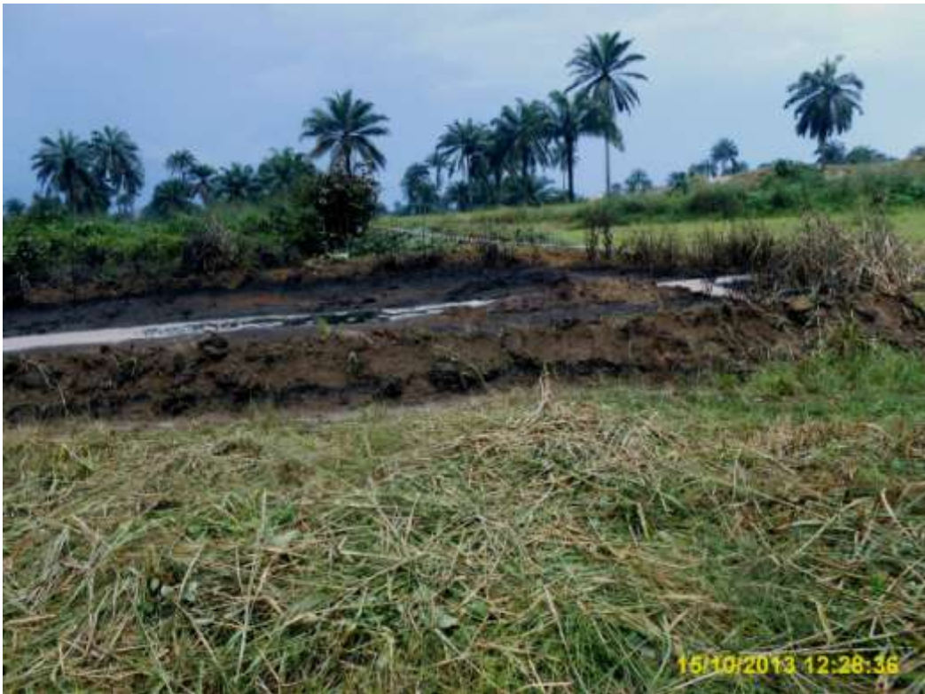
Overview: Part of spill/fire impact on 28" Trans Niger Pipeline (near Patrick Waterside manifold) right of way at Bodo-city. Picture was taken during Joint Investigation of 15 th October 2013.
