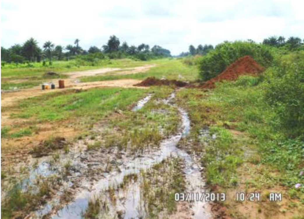
Overview: Part of spill impact on 36" Rumuekpe-Nkpoku Trans Niger Pipeline right of way at Omuigwe-Aluu. Picture was taken during Joint Investigation of 3 rd November 2013.
