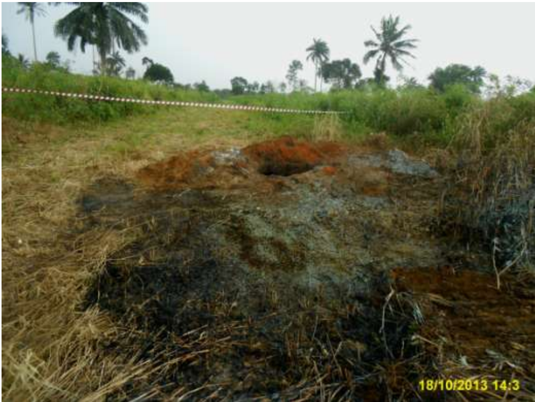
Overview: Part of spill/fire impact on 24" Nkpoku - Bomu Pipeline right of way at Biara. Picture was taken during Joint Investigation of 18 th October 2013.
