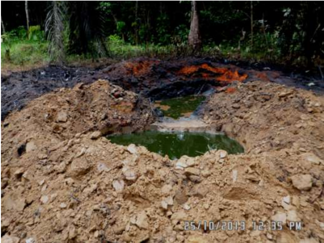
Overview: Part of spill/fire impact on 24" Nkpoku - Bomu Trans Niger Pipeline right of way at Biara/Kpите. Picture was taken during Joint Investigation of 25 th October 2013.
