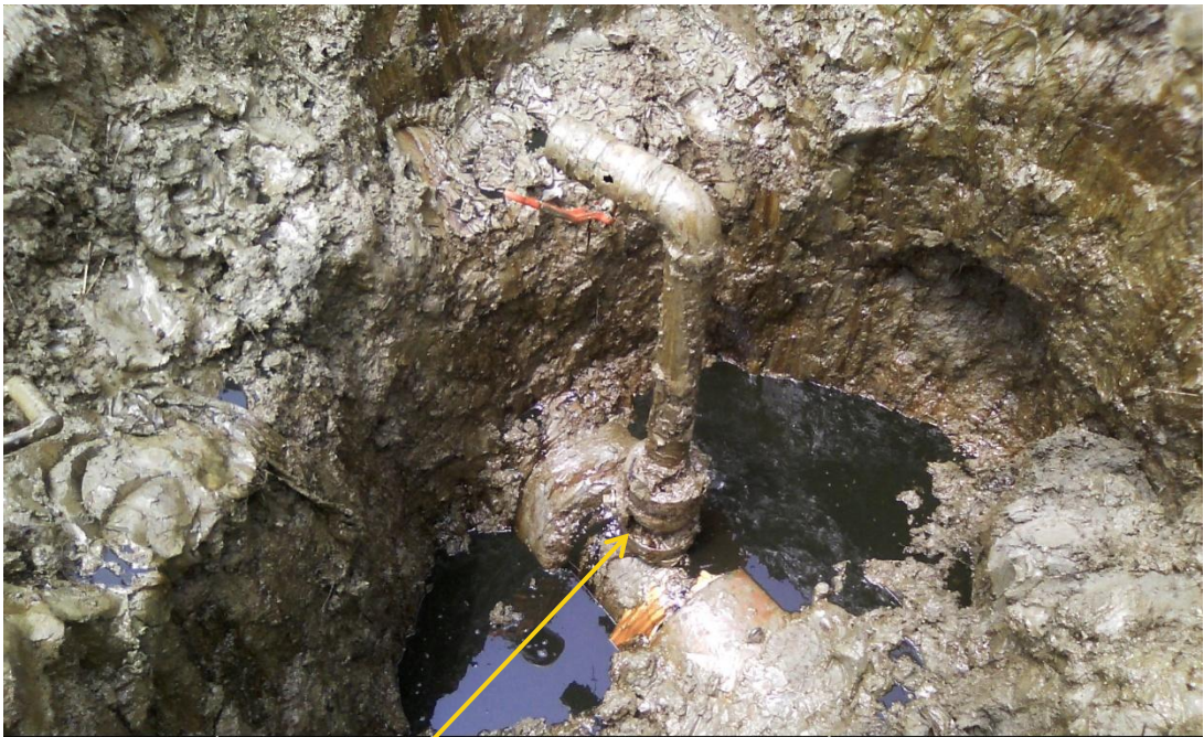
Overview: Part of spill impact on 14" Okordia - Rumuekpe Pipeline at Akaramini. Picture was taken during Joint Investigation of 23 rd October 2013.
