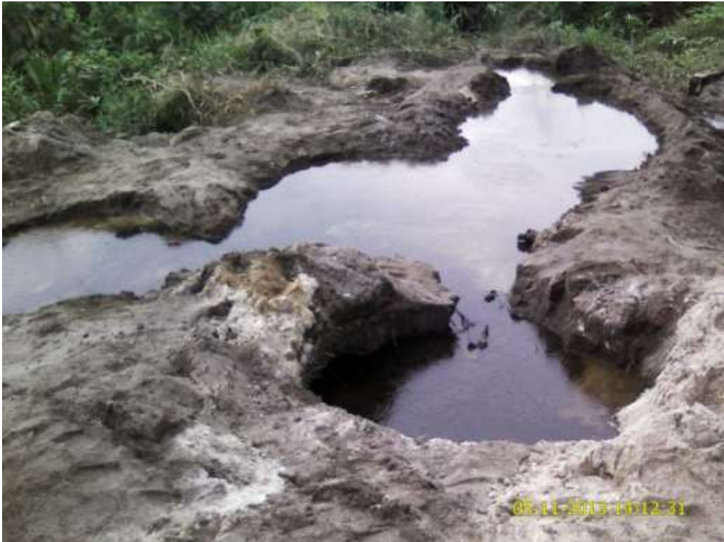
Overview: Part of spill impact on 28" Nkpoku-Bomu Pipeline right of way at Gio. Picture was taken during Joint Investigation of 5th November 2013.
