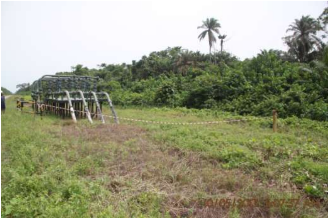
Overview: Part of spill impact on Yokri Manifold7 Low Pressure1 line right of way at Sokebolou. Picture was taken during Joint Investigation of 10 th May 2013.
