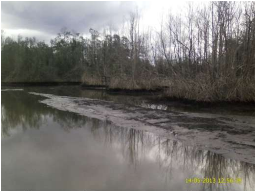
Overview: Part of spill impact on 30" Nembe Creek pipeline right of way at Boro (Kula). Picture was taken during Joint Investigation of 14 th May 2013.
