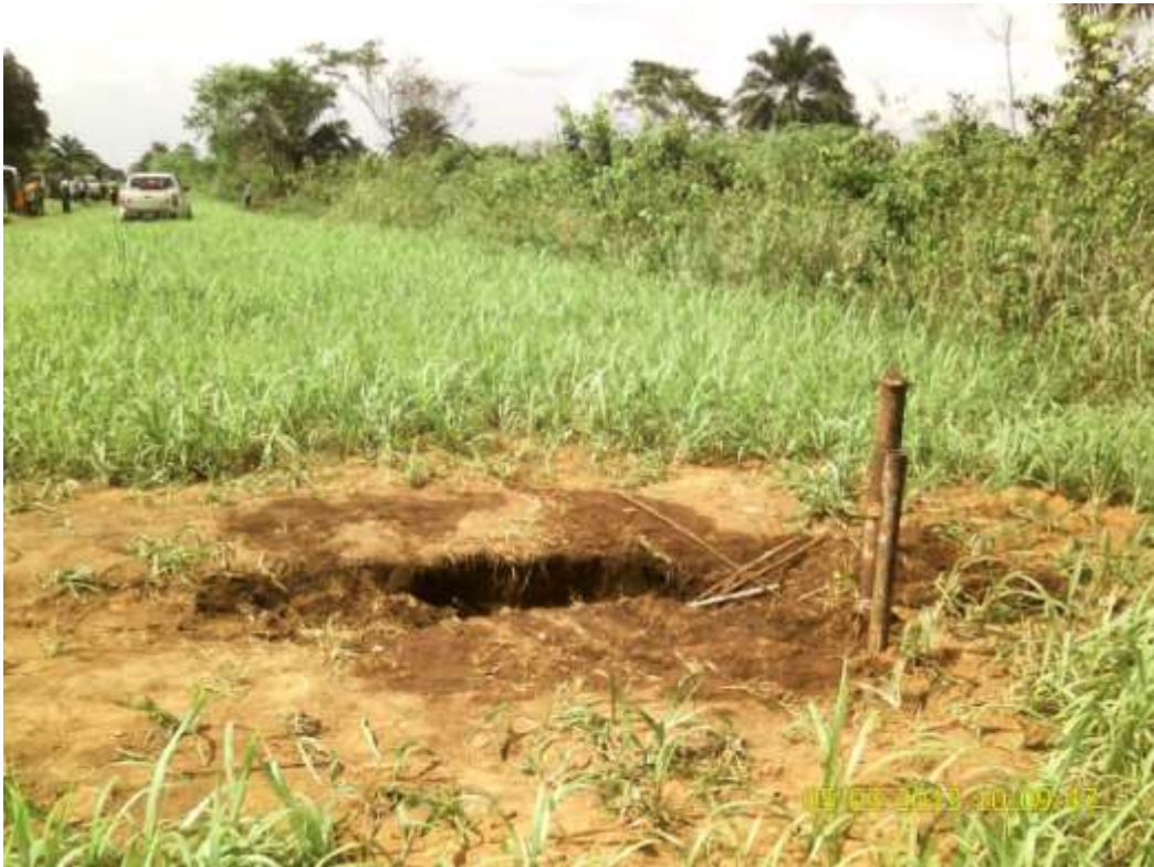
Overview: Part of spill impact Hacksaw cut on 8" Assa-Rumuekpe pipeline right of way at Awara. Picture was taken during Joint Investigation of 5 th March 2013.
