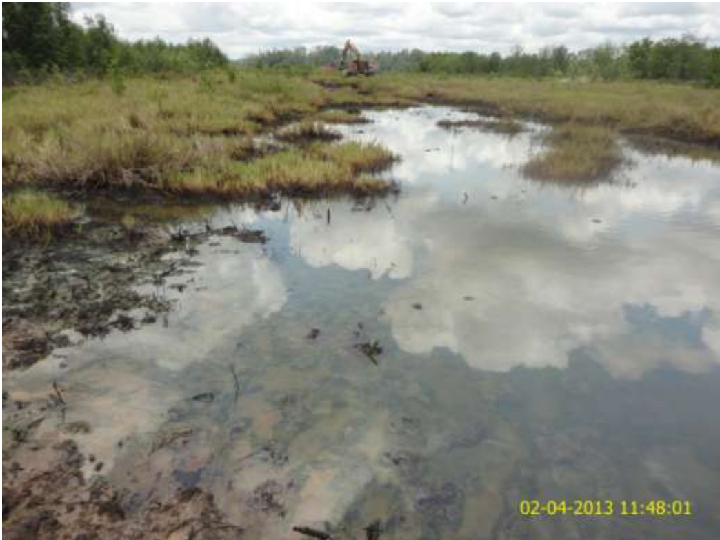
Overview: Part of spill impact on 24" Nembe Creek Trunkline right of way at Aberedo-A. Picture was taken during Joint Investigation of 2 nd April 2013.
