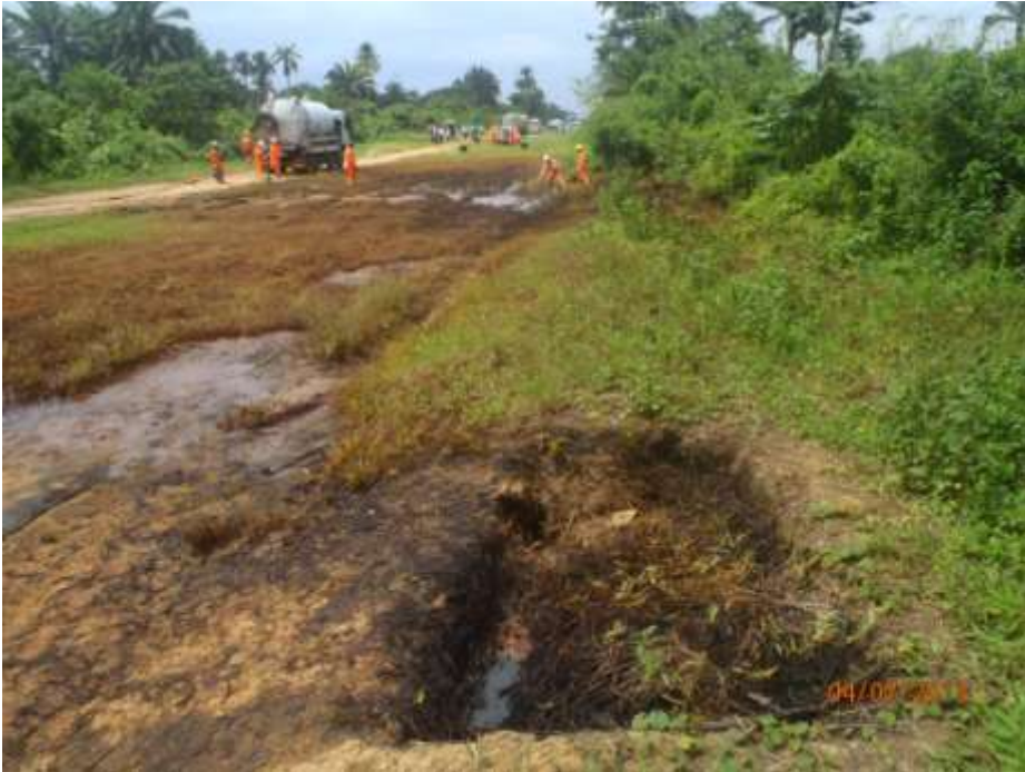
Overview: Part of spill impact on 36" Nkpoku-Bomu pipeline right of way at Rumuowegwu. Picture was taken during Joint Investigation of 4 th July 2013.
