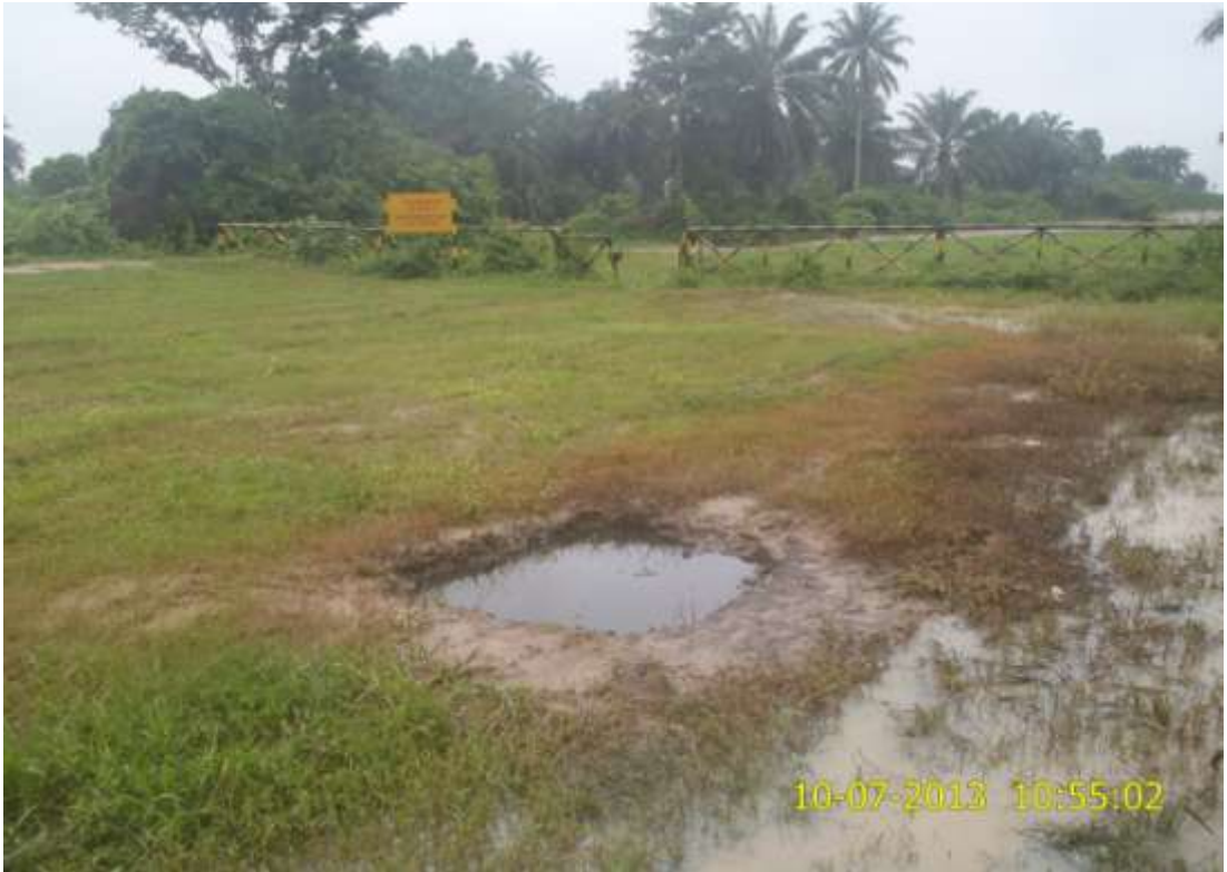
Overview: Part of spill impact on 24" Nkpoku-Bomu pipeline right of way at Rumuoegwu-Eneka. Picture was taken during Joint Investigation of 10 th July 2013.
