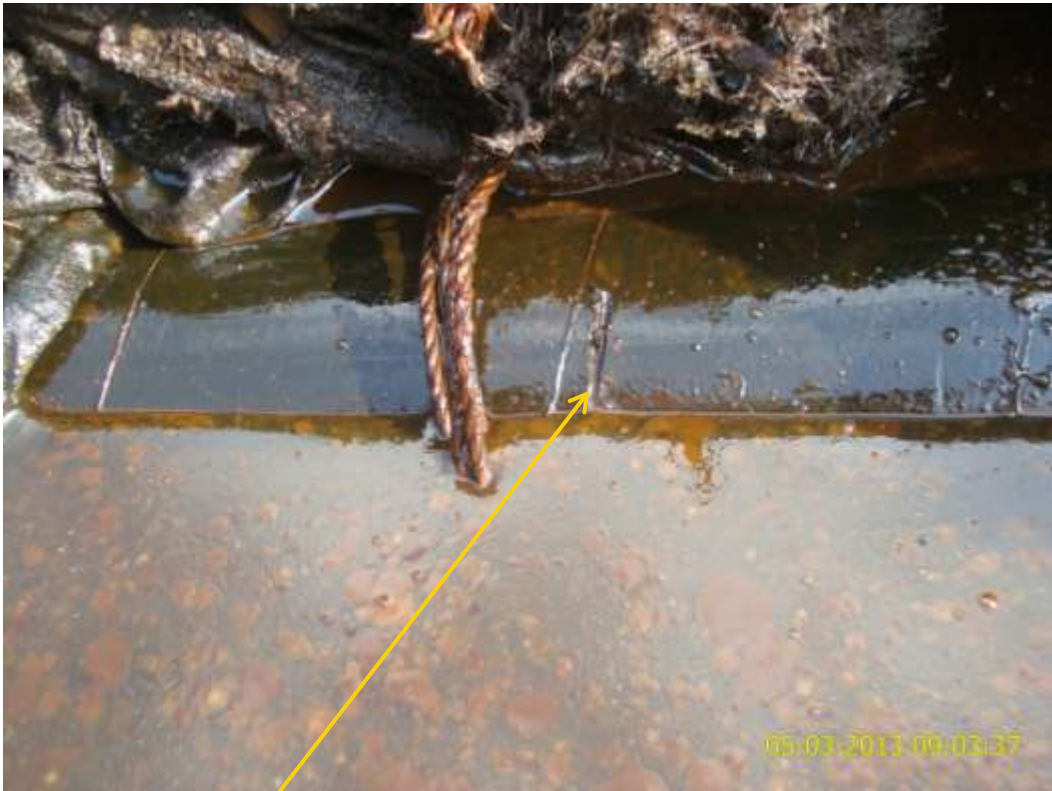
Close up: Hacksaw cut on 4" Awoba North West Well L & S flowlines at Boro. Picture was taken during Joint Investigation of 5 th March 2013.
