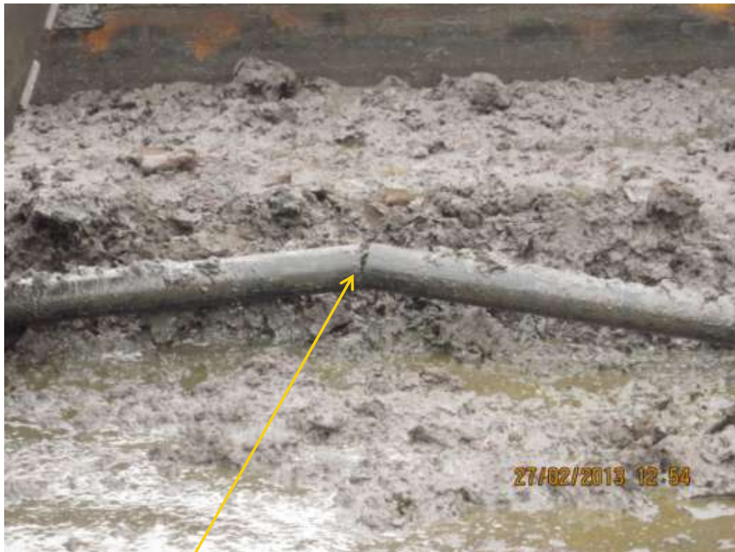
Close up: Cut flowline section on Nembe 2 Well17S flowline at Nembe. Picture was taken during Joint Investigation of 27 th February 2013.
