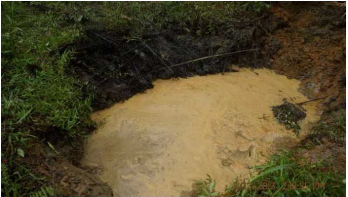
Overview: Part of spill impact on 20" Otumara - Escravos Pipeline right of way at Ogidigben. Picture was taken during Joint Investigation of 11th December 2013.
