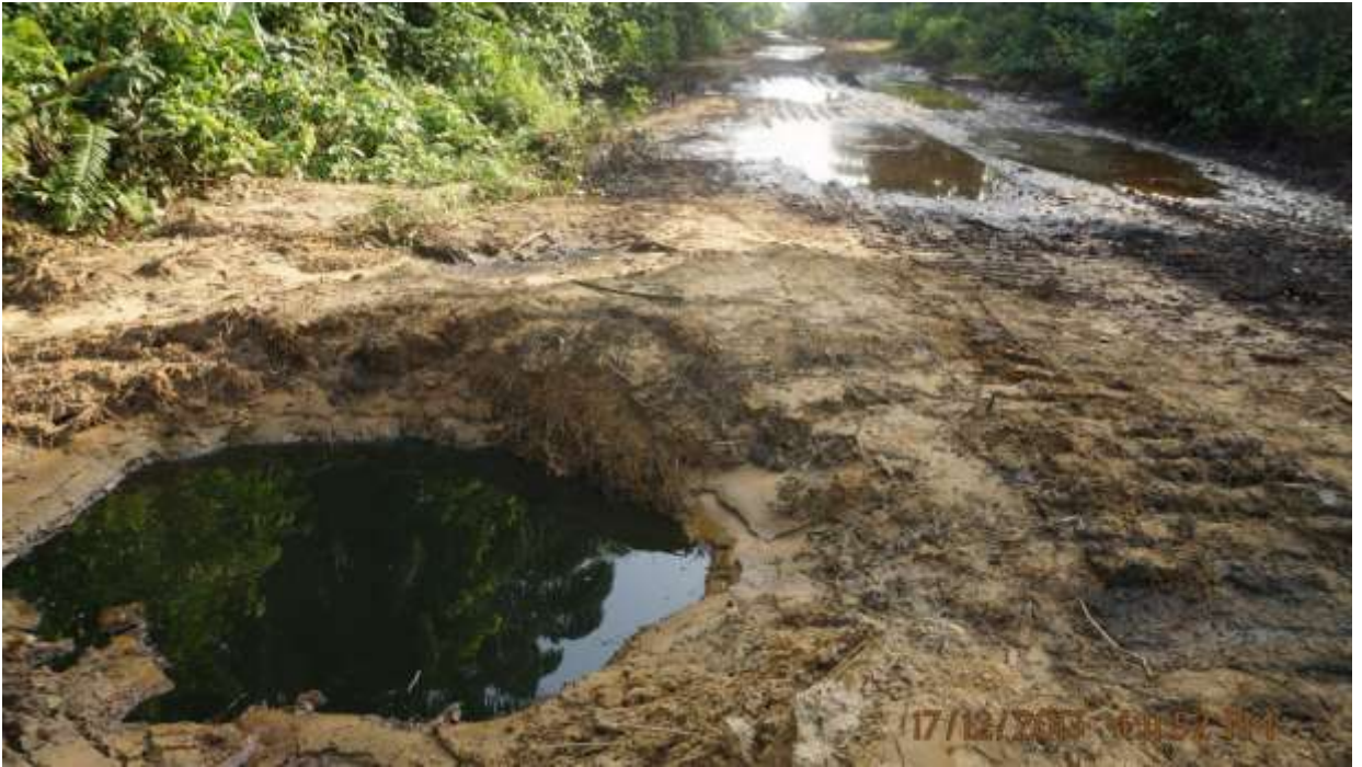
Overview: Part of spill impact on 20" Otumara – Escravos Pipeline right of way at Adjudaibo. Picture was taken during Joint Investigation of 17 th December 2013.
