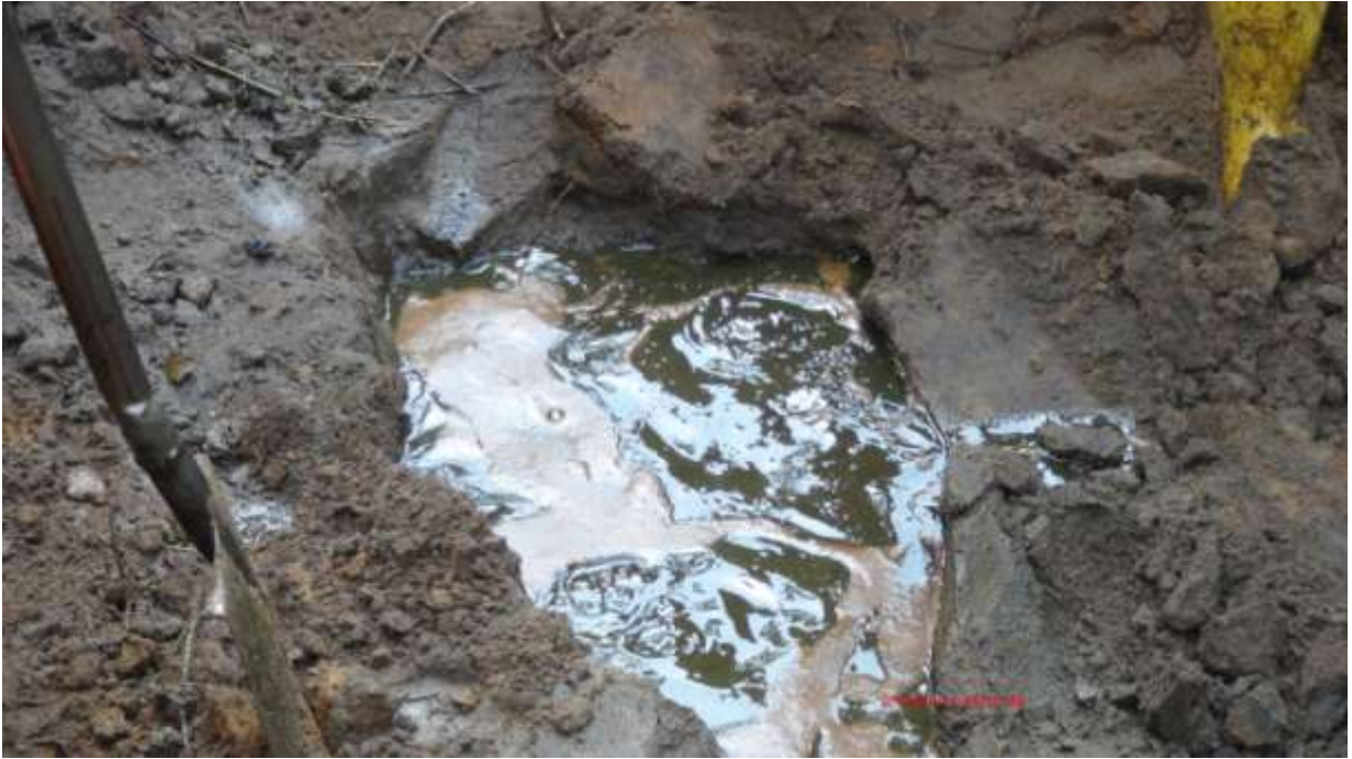
Overview: Part of spill impact on 4" Well69S Flowline right of way at Umuokwa. Picture was taken during Joint Investigation of 3rd January 2014.
