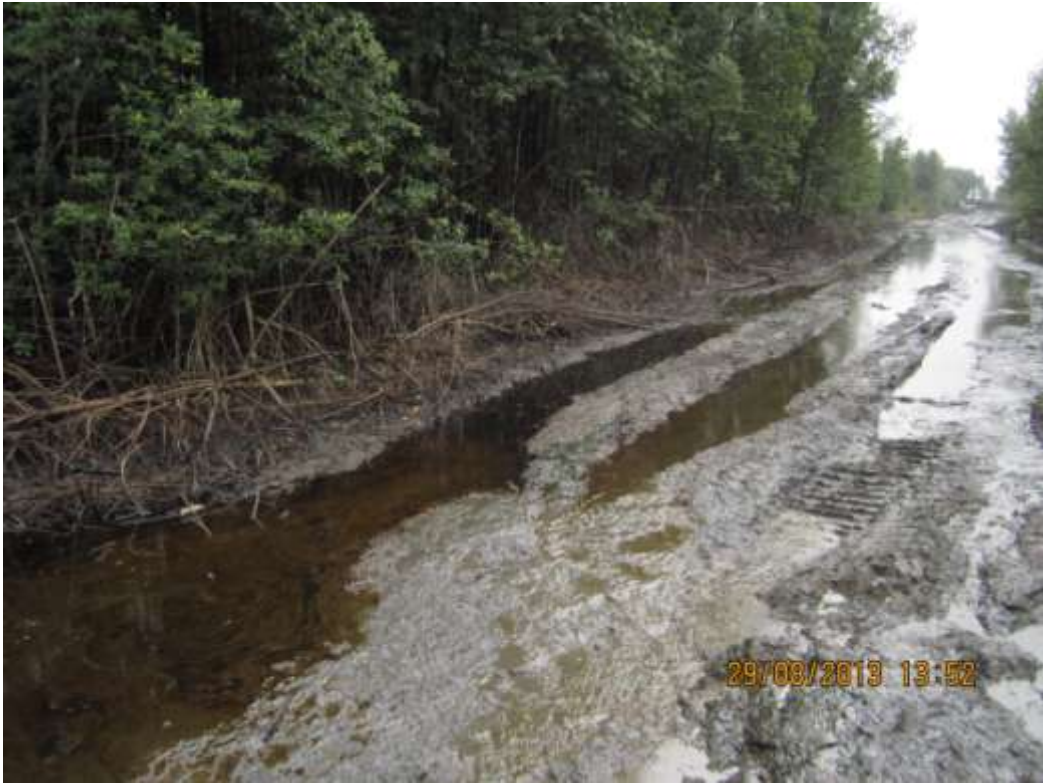
Overview: Part of spill impact on 10" Ekulama1 – Sanbarth Pipeline right of way at Ekulama. Picture was taken during Joint Investigation of 29th August 2013.
