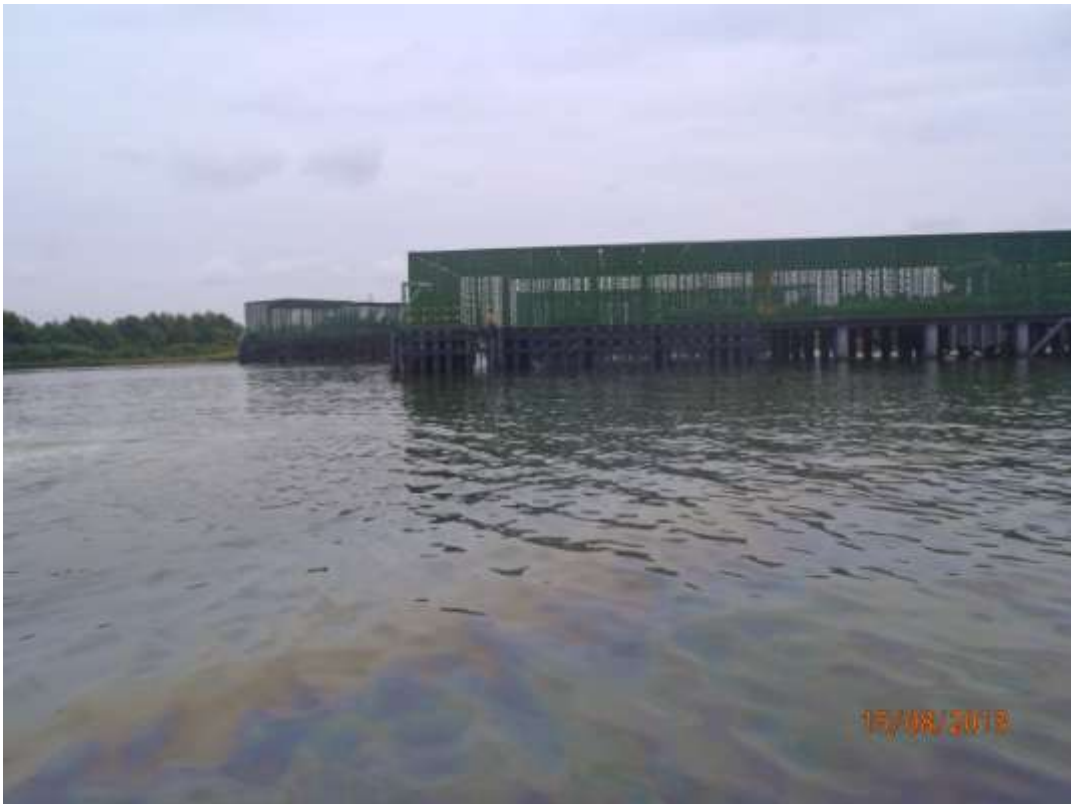
Overview: Part of spill impact on 24" Cawthorne-Channel loopline manifold right of way at Ilomaturu. Picture was taken during Joint Investigation of 15 th August 2013.
