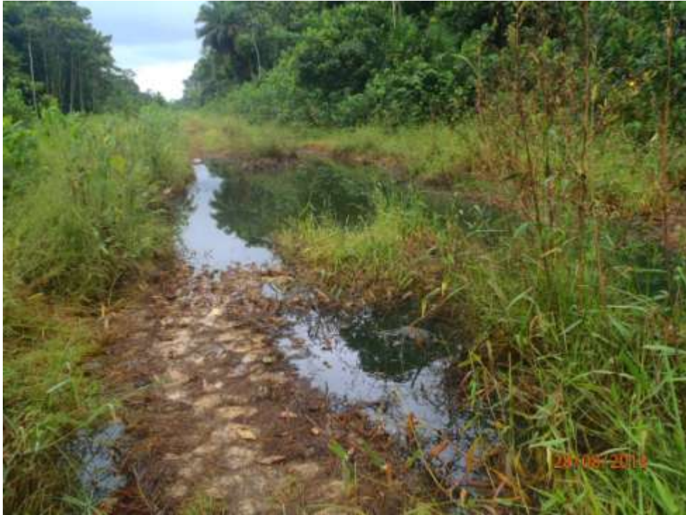
Overview: Part of spill impact on 16" Nun River – Kolocreek pipeline right of way at Igiebiri. Picture was taken during Joint Investigation of 28 th August 2013.
