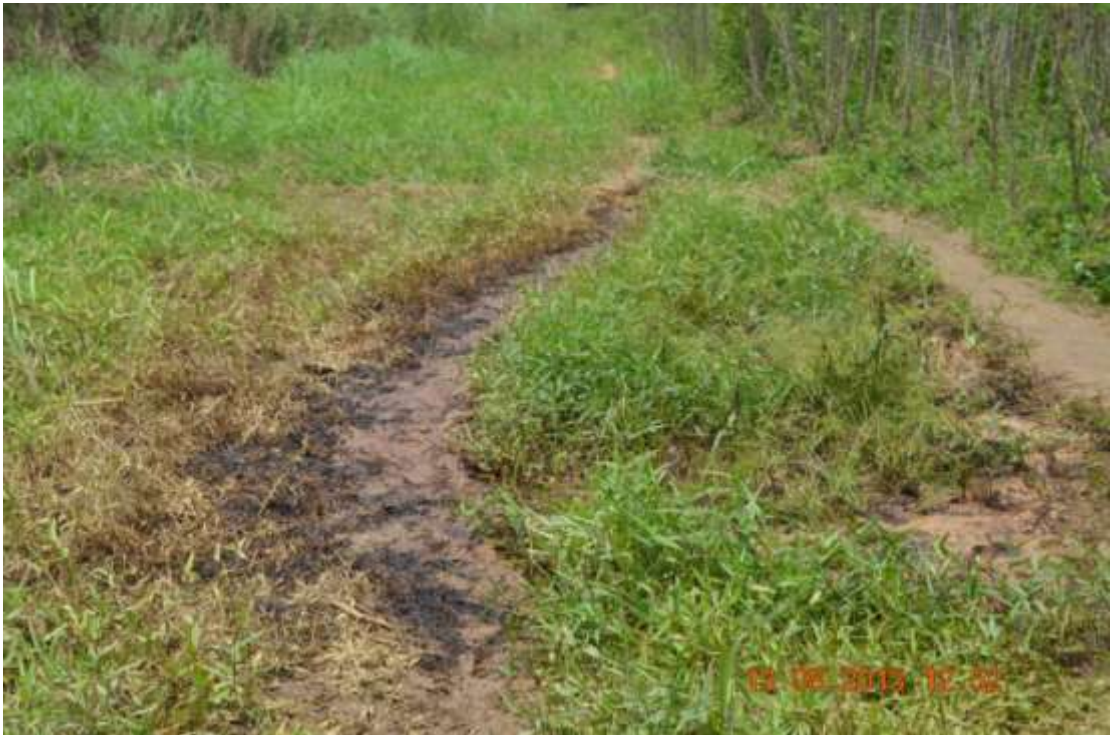
Overview: Part of spill impact on 14" Okordia-Rumuekpe pipeline right of way at Ikarama. Picture was taken during Joint Investigation of 13 th August 2013.
