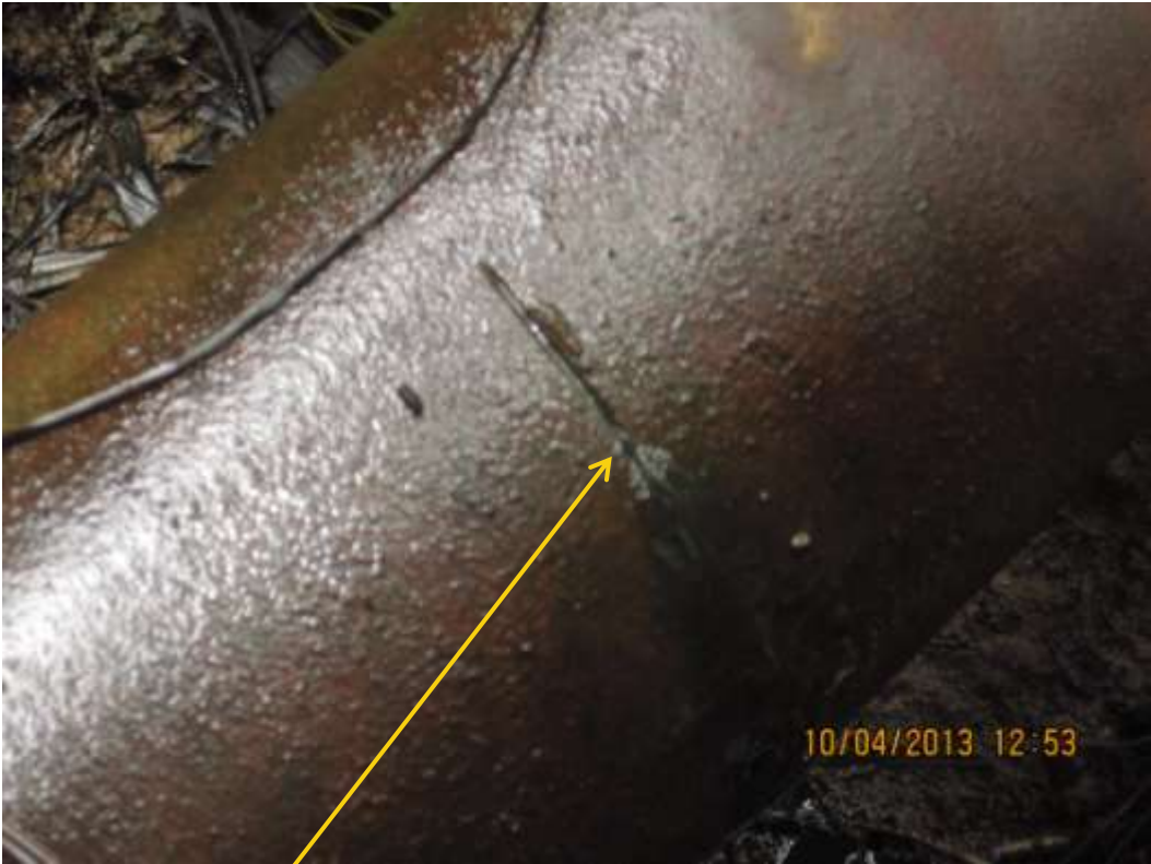
Close up: Hacksaw cut on 4" Adibawa Well10S flowline at Edagberi. Picture was taken during Joint Investigation of 10 th April 2013.
