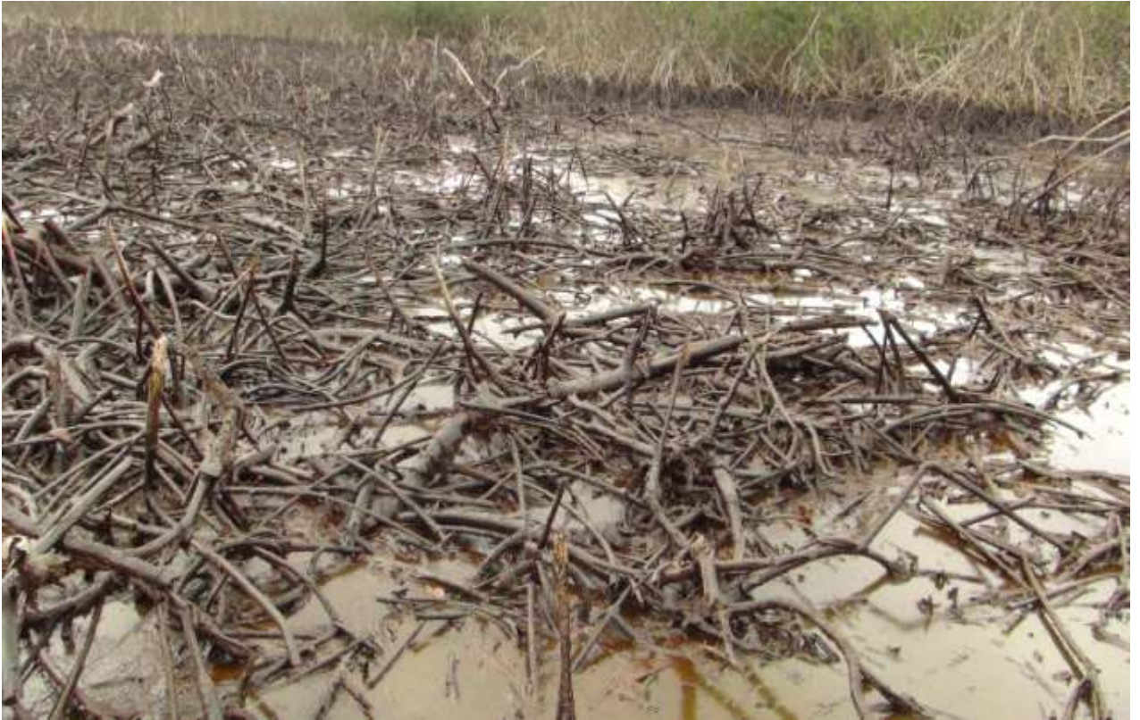
Overview: Part of spill impact on Cawthorne Channel 1 Well 49L at Cawthorne Channel. Picture was taken during Joint Investigation of 19th Sept. 2012.
