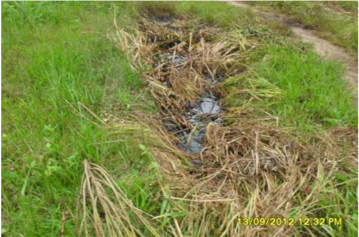
Overview: Part of spill impact on 16'' Uzere-Eriemu Pipeline at Iyede. Picture was taken during Joint Investigation of 13 th Sept. 2012.
