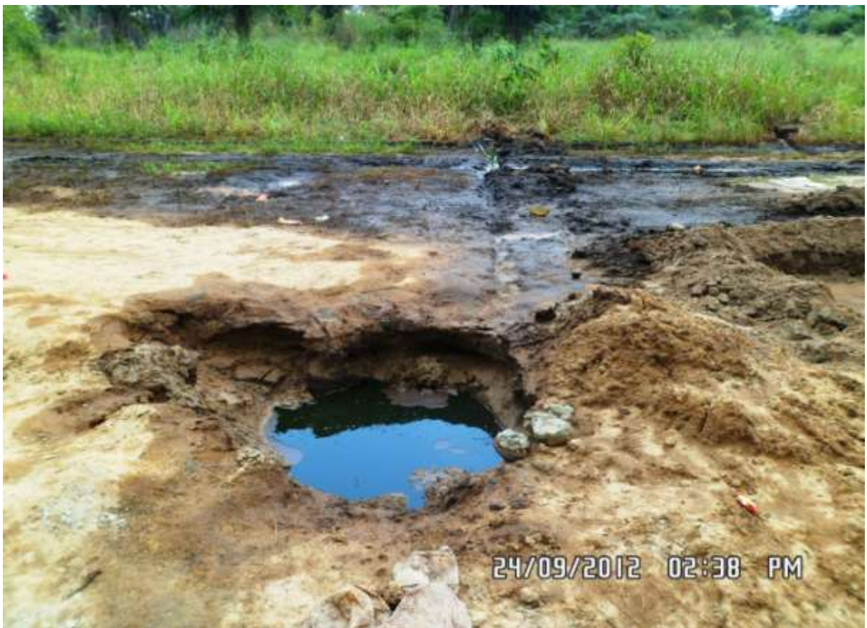
Overview: Part of spill impact on 28" Nkpoku - Bomu Pipeline at Gio. Picture was taken during Joint Investigation of 24 th Sept. 2012.
