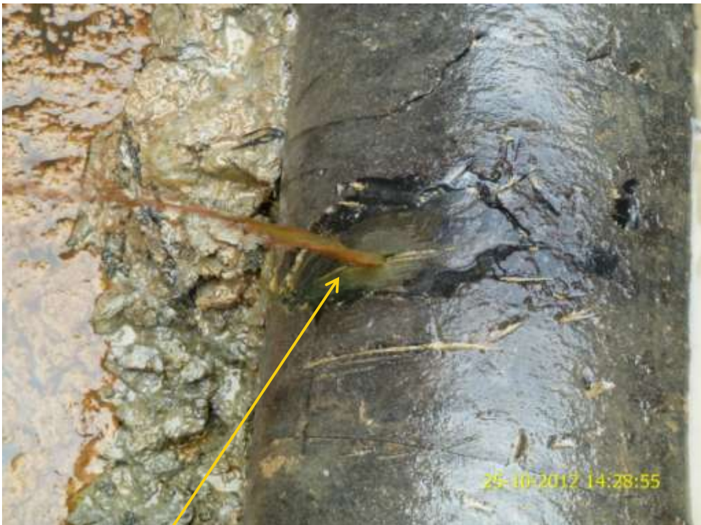
Close up: Hacksaw cut on 10" Nun River delivery line at Ekowe. Picture was taken during Joint Investigation of 25 th October 2012.
