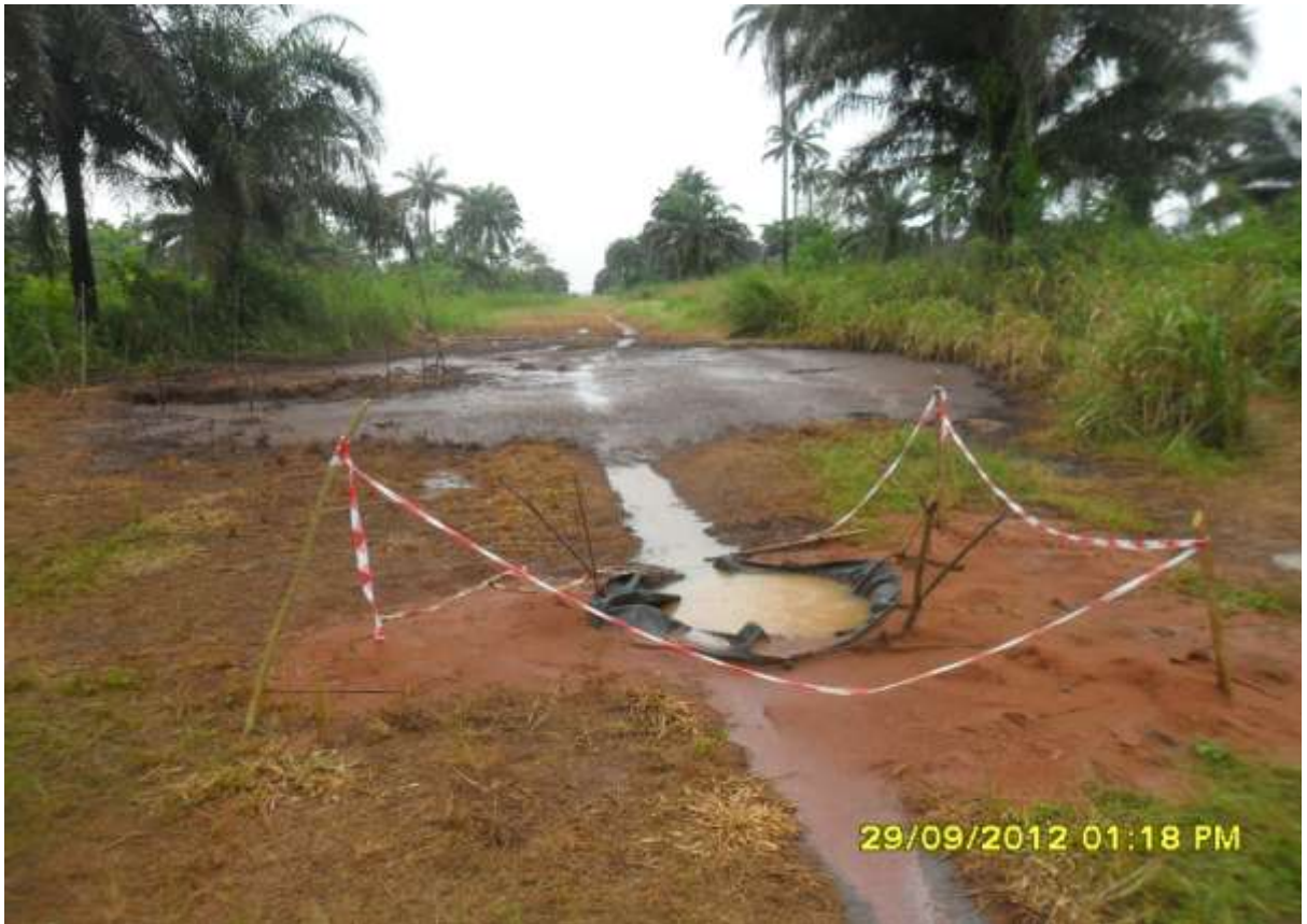
Overview: Part of spill impact on 16'' Egbema-Assa Pipeline At Umudike. Picture was taken during Joint Investigation of 29 th Sept. 2012.
