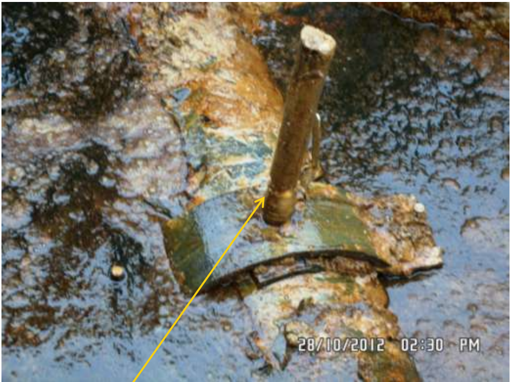
Close up: Illegal fitting on 12" Imo River 2 pipeline at Umuedeokwara. Picture was taken during Joint Investigation of 28 th October 2012.
