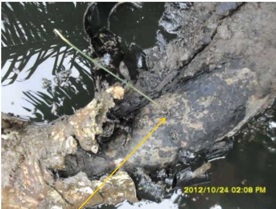
Close up: Spill due to pinhole on Otumara Well20L flowline at Ugboegungun. Picture was taken during Joint Investigation of 24 th October 2012.
