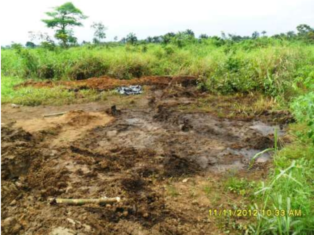
Overview: Part of spill impact on 28" Nkpoku-Bomu pipeline right of way at Gio. Picture was taken during Joint Investigation of 11 th November 2012.
