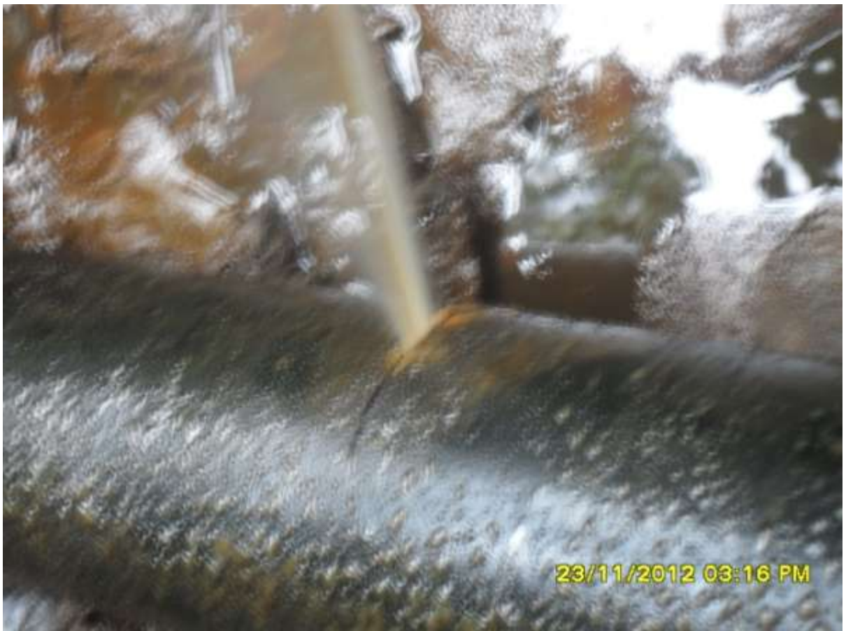
Close-up: Hacksaw cut on Imo River Well 64S/L Flowline at Owaza. Picture was taken during Joint Investigation of 23 rd Nov. 2012.
