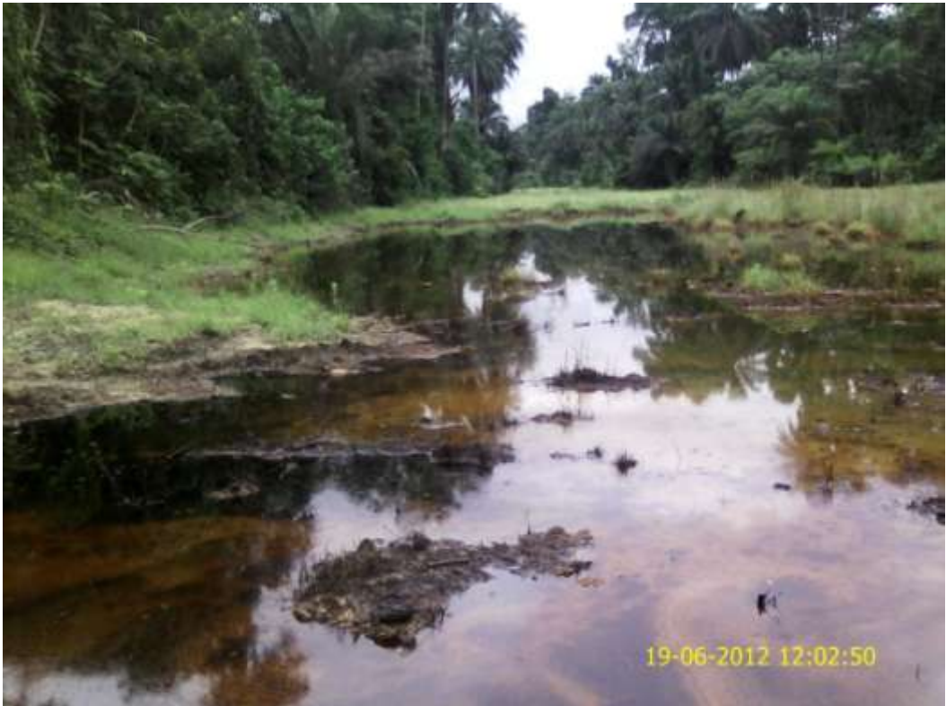
Overview: Part of spill impact on 14" Okordia-Rumuekpe pipeline right of way at Ikarama. Picture was taken during Joint Investigation of 19 th June 2012.
