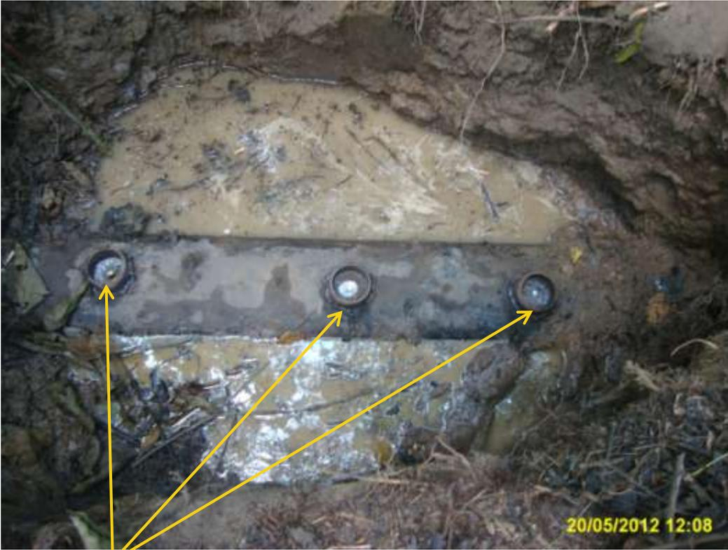
Close up: Illegal fittings on 12" Imo river pipeline at Uzuaku. Picture was taken on 20<sup>th</sup> May 2012.
