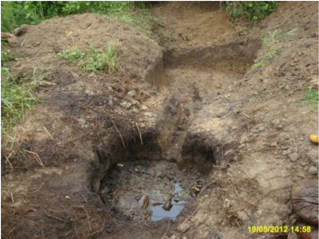
Overview: Part of spill impact on 12" Imo River1 pipeline right of way at Uzuaku. Picture was taken during Joint Investigation of 19 th May 2012.
