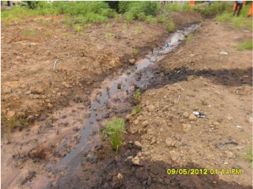
Overview: Part of spill impact on 28" Bomu-Bonny pipeline at K-Dere. Picture was taken during Joint Investigation of 9 th May 2012.
