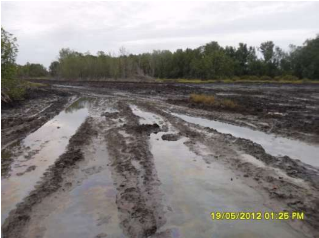
Overview: Part of spill impact 10" Ekulama1-Sanbarth pipeline right of way at Ekulama1. Picture was taken during Joint Investigation of 19 th May 2012.
