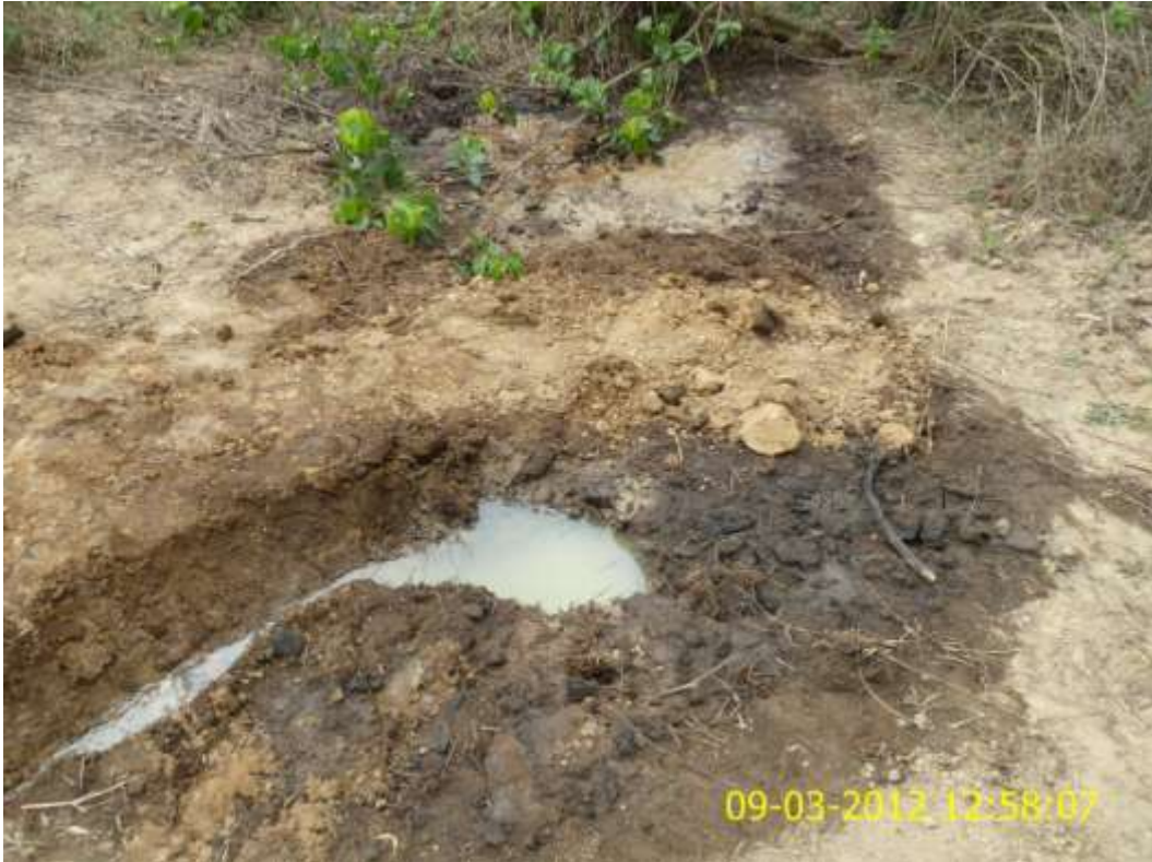
Overview: Part of spill impact on 24" Nkpoku-Bomu pipeline right of way at Egballor. Picture was taken during Joint Investigation of 9 th March 2012.
