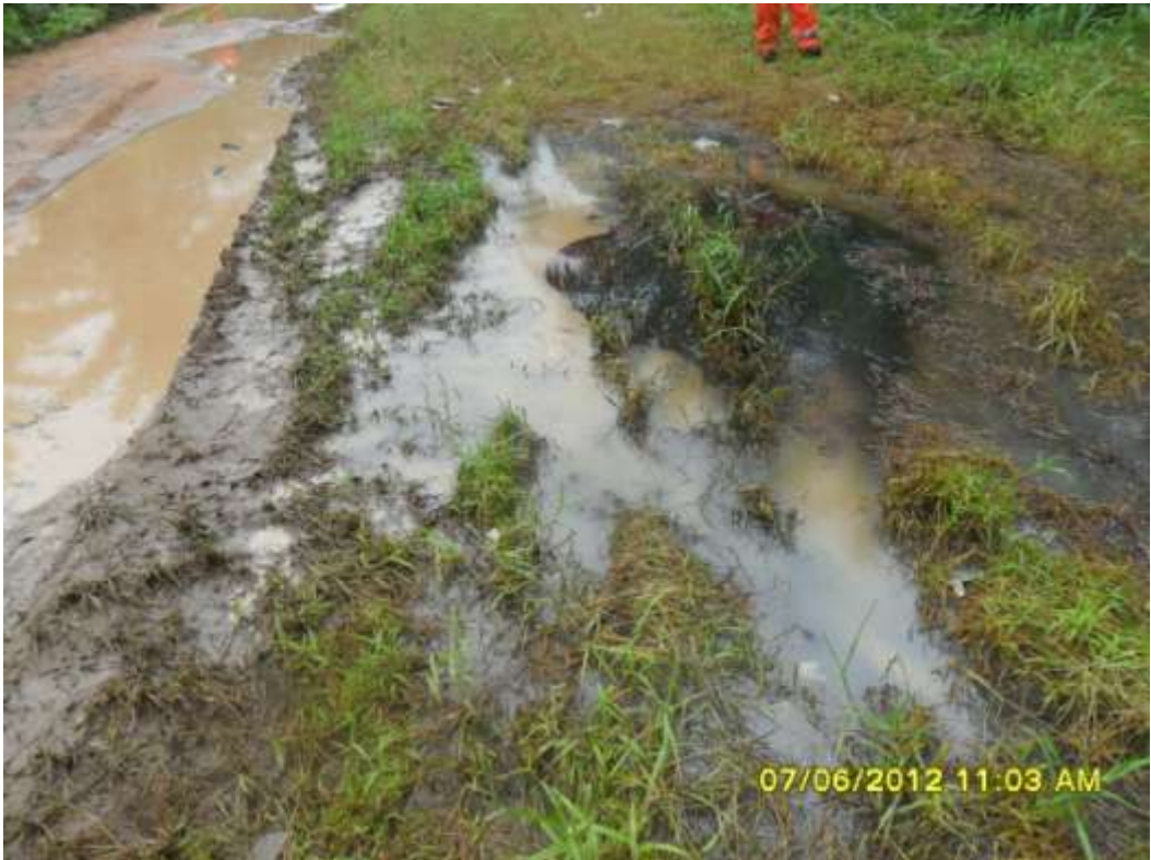
Overview: Part of spill impact on 18" Assa-Rumuekpe pipeline right of way at Omudioga. Picture was taken during Joint Investigation of 7 th June 2012.
