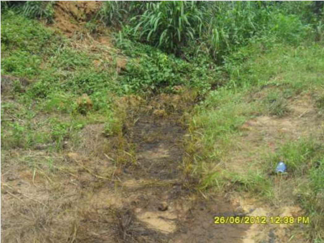
Overview: Part of spill impact on 24" Npoku-Bomu trunkline right of way at Botem. Picture was taken during Joint Investigation of 26 th June 2012.
