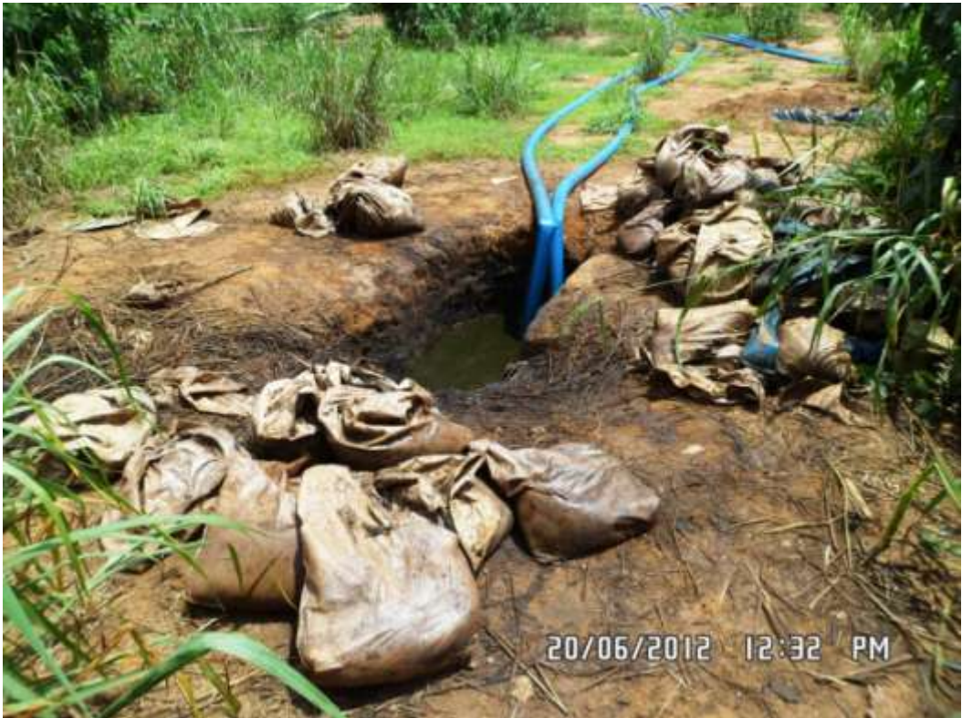
Overview: Part of spill impact on 24" Npoku-Bomu Trans Niger Pipeline right of way at Nonwa. Picture was taken during Joint Investigation of 20 th June 2012.
