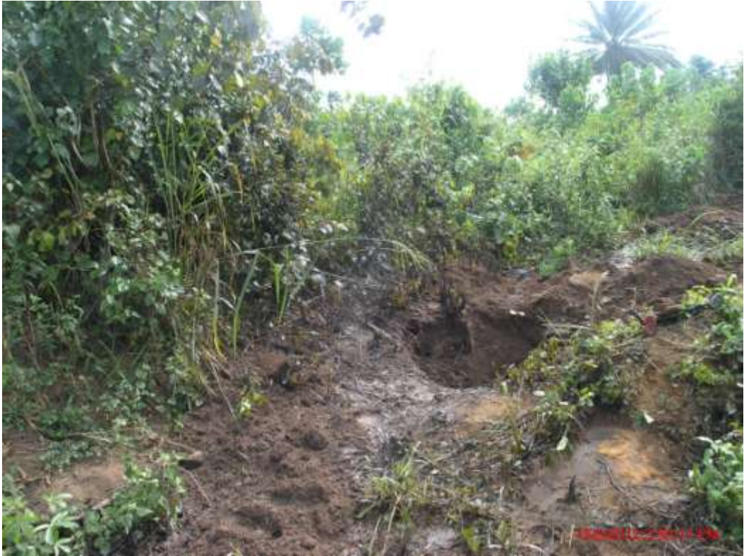
Overview: Part of spill impact on 24" Nembe Creek Trunkline right of way behind Seگو Manifold. Picture was taken during Joint Investigation of 27 th May 2012.
